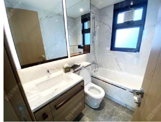
Toilet With Better Ventilation
